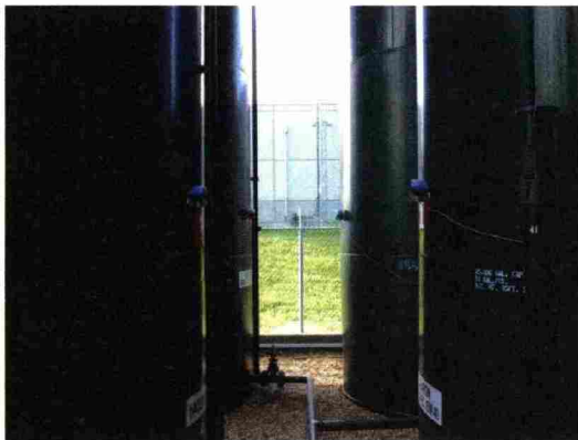
Tank level monitoring systems, such as those from TankLink, ensure the correct amount of product is delivered.
